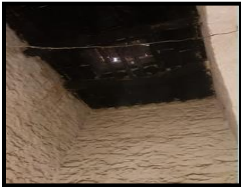
Figure: 22(author) Roof ventilator which can be opened or closed when required. Even seasonal wise, in rainy it can be closed
