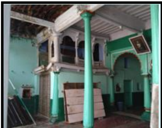
Figure: 24(author) Kacheri, Hypostyle column with separate ladies seating area covered with jail work. Parda system followed at that time.
