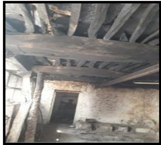
Figure: 19(author) servant's area, Rough finished roof structure.
