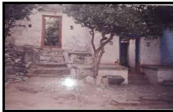
Figure: 8(author) Entrance katta on both the sides with common wall between two houses. Entrance door height and width is also small.
