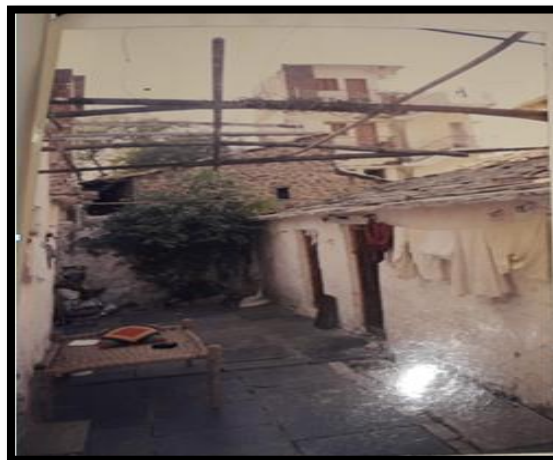
Figure: 9(author) Courtyards connecting all rooms through door openings as windows were not provided. Attached houses with common wall
