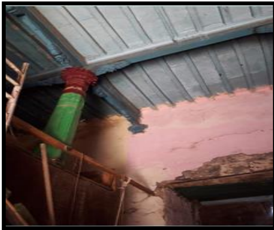
Figure: 18(author) Fine finished double height entrance Jhalji.
