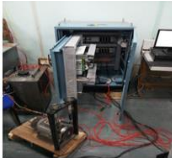
Figure 3: Micro-grid prototype with various loads connected to the PMU
